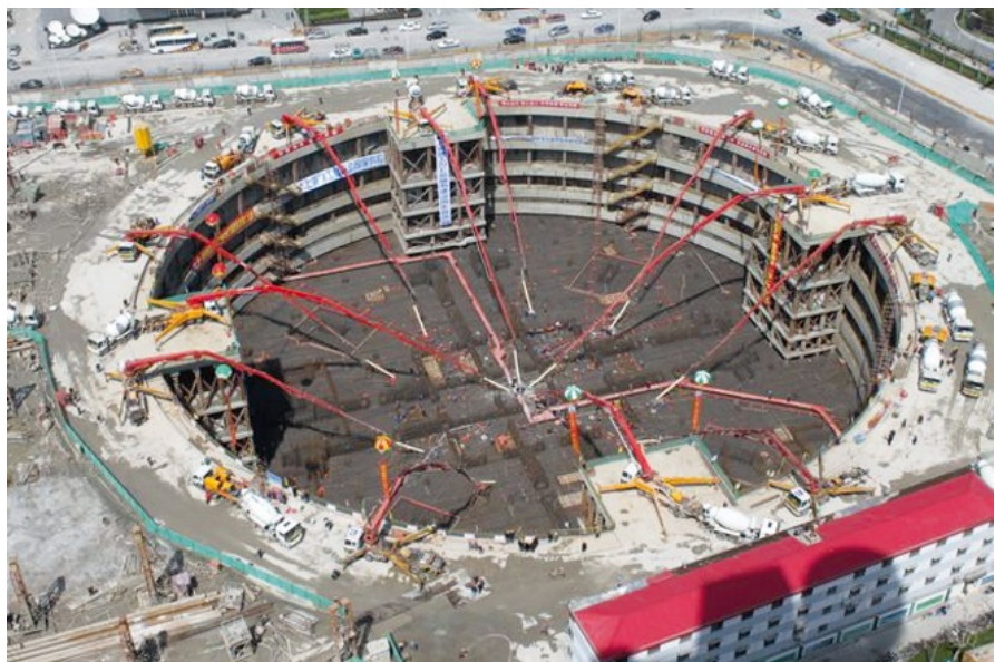
Figure 2. Shanghai Tower underground construction site. Retrieved from ZWP Ingenieur-AG [8].
