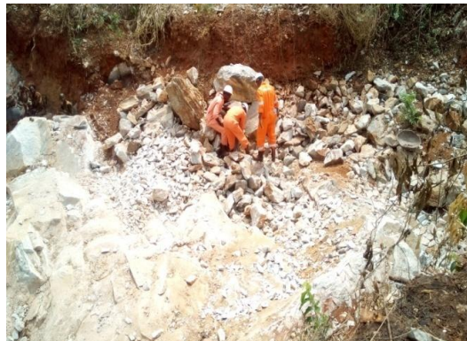
Fig. 6a. Field photograph showing small-scale marble mining pit at Igue Oke
