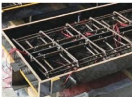
(a) Steel-concrete combination beams-PBL
