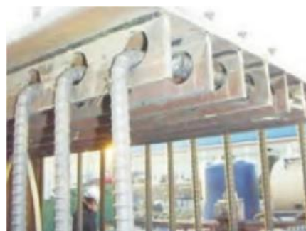
(b) Steel-concrete bonding section-PBL
